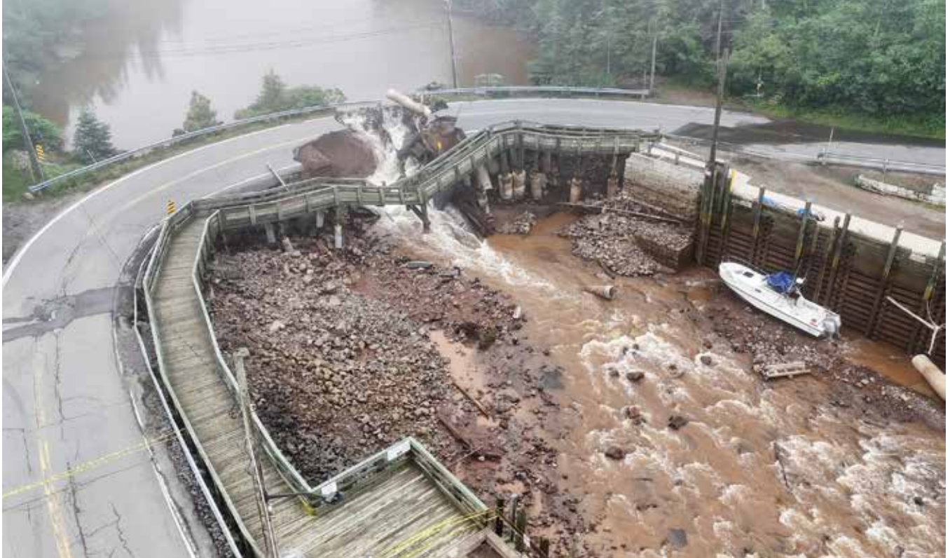
Recreated illustration of damage from Halls Harbour flood in July 2024. (Communications Nova Scotia)
